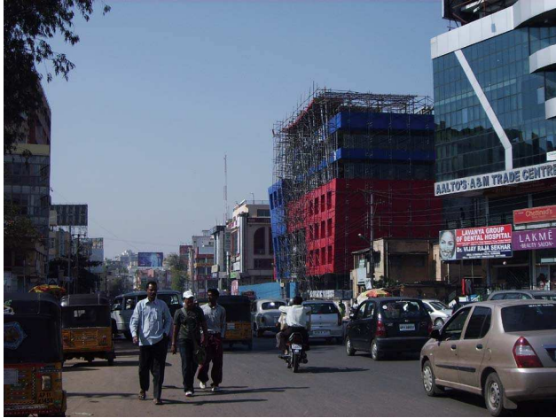
Figure 3: Construction work on Himayatnagar Main Road. Own source, Feb. 2008.
